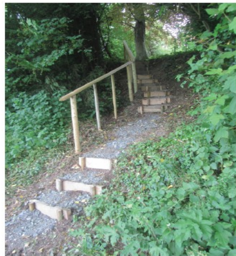
The footpath beside Raglands has been reinstated on its correct alignment.
