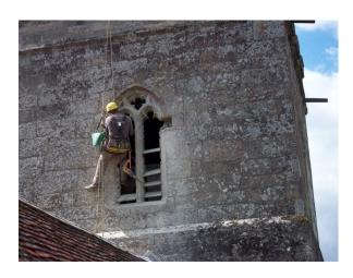
By securing their ropes on the top of the tower, and using special karabiners, they are able to descend to the appropriate spot and stop. They then have both hands free to work while hanging in a seat from the rope. When finished, they use the karabiner to ascend to the start point.
